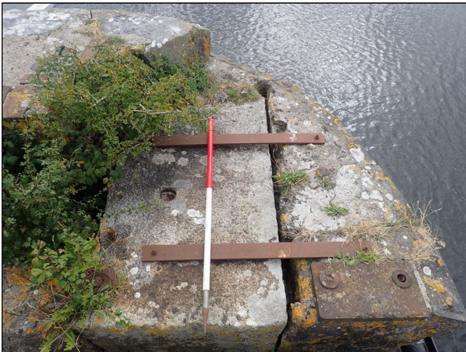
Plate 32: South-facing view of historic repair work to consolidate coping on the southwest side of the structure (1m scale).
