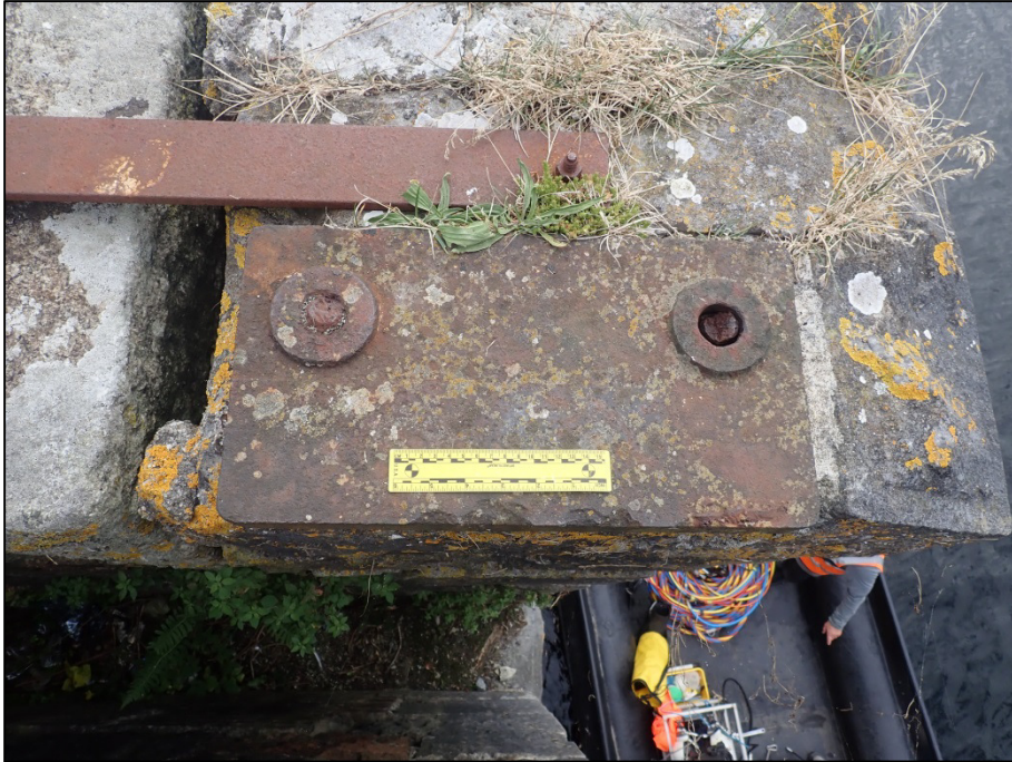
Plate 27: Detail shot of iron-plate secured to coping on south side of pier structure, top of Pier Number 1 (150mm scale).
