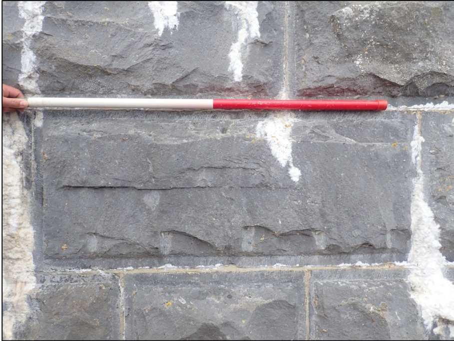
Plate 11: Example shot of rock-faced limestone ashlar used in the construction of the pier walls (1m scale); shot taken on western façade of Pier Number 3.
