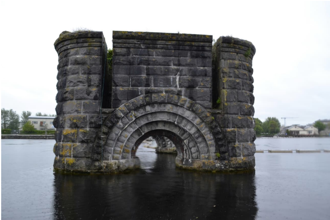
Plate 13 No. 1 pier- west facing elevation. Note rebates for the drawbridge.
