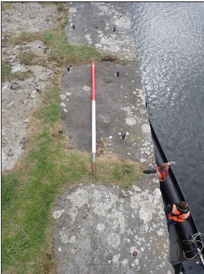
Plate 26: South-facing view of coping on west side of Pier Number 1 showing remnants of fixing-points protruding from the masonry (1m scale).
