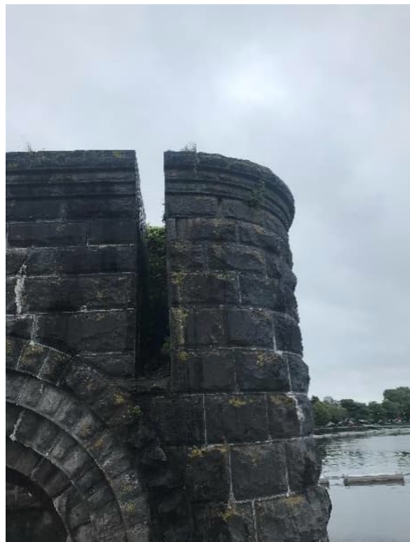
Photo No.4 – Damage noted to Pier No.1
