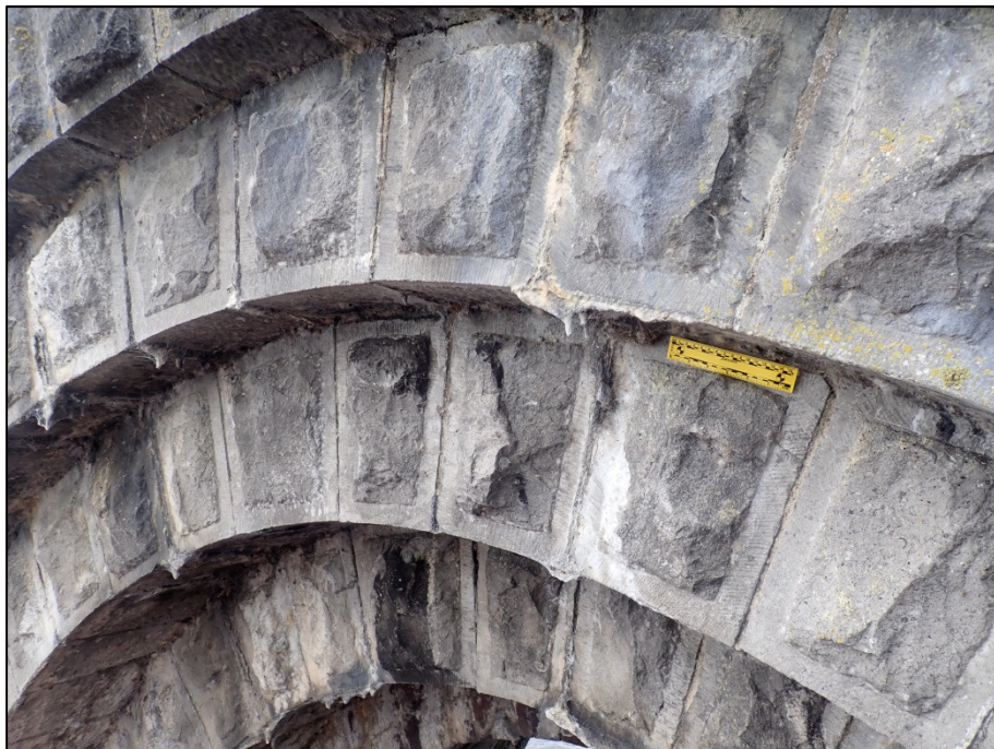
Plate 18: Detail shot of the masonry used in the tiered arch-rings that form the Romanesque style archways located on Pier Numbers 1 and 2 (150mm scale).
