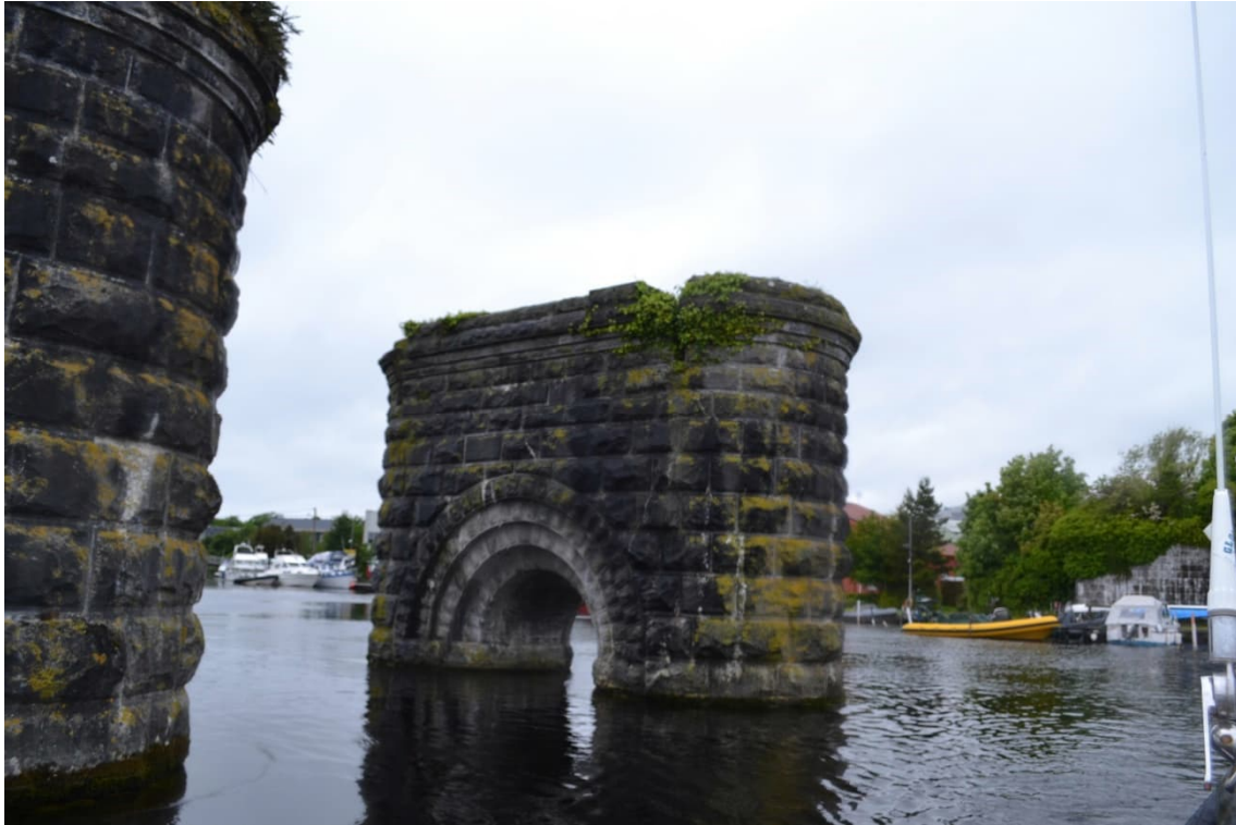
Plate 15 No. 1 pier – rebates on east facing elevation.
