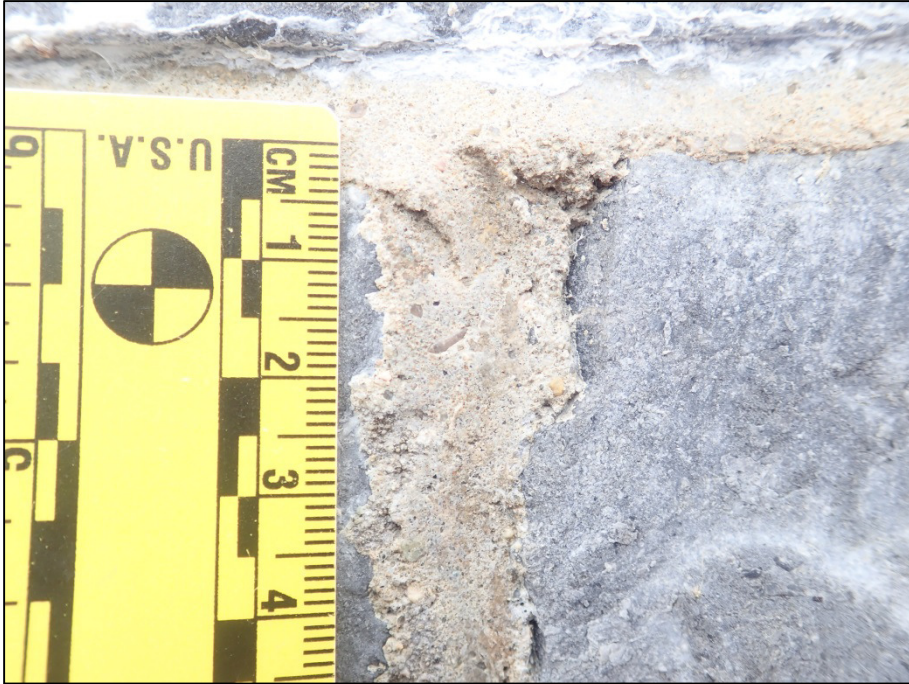
Plate 13: Detail shot showing mortar used to bond the masonry together (45mm scale).
