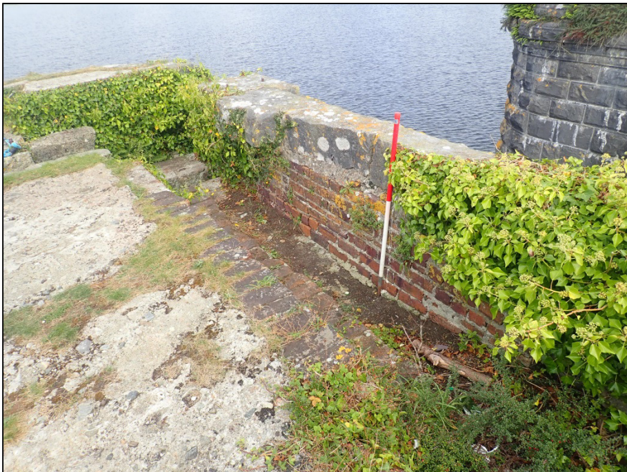
Plate 28: NNE-facing view of top of Pier Number 1 showing use of brickwork on inside of pier wall (1m scale).
