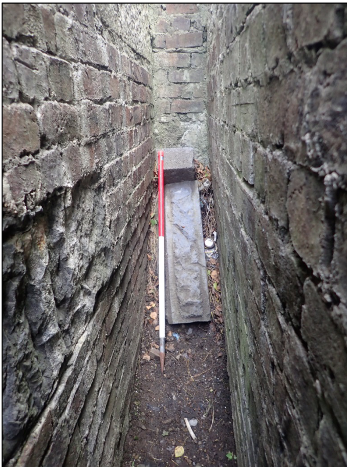
Plate 30: Example shot showing construction of side walls within recess/ slot (north slot) on west side of Pier Number 1.
