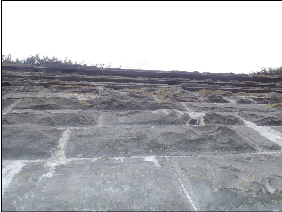
Plate 15: Example shot of oversail coping present at the top of Pier Number 3, shot taken on west side of structure.
