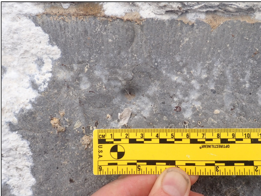
Plate 14: Detail shot of the cone-shaped 'pincer holes' located top/centre of each masonry block (100mm scale).
