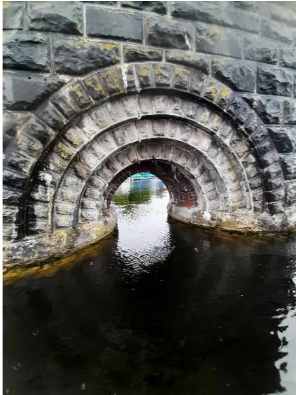
Photo No.4 – Arch rings to Pier No. 1
