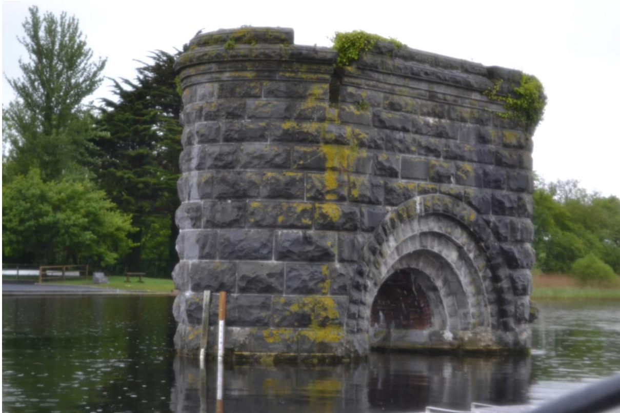
Plate 17 No. 1 pier- damage to string course on east facing elevation.
