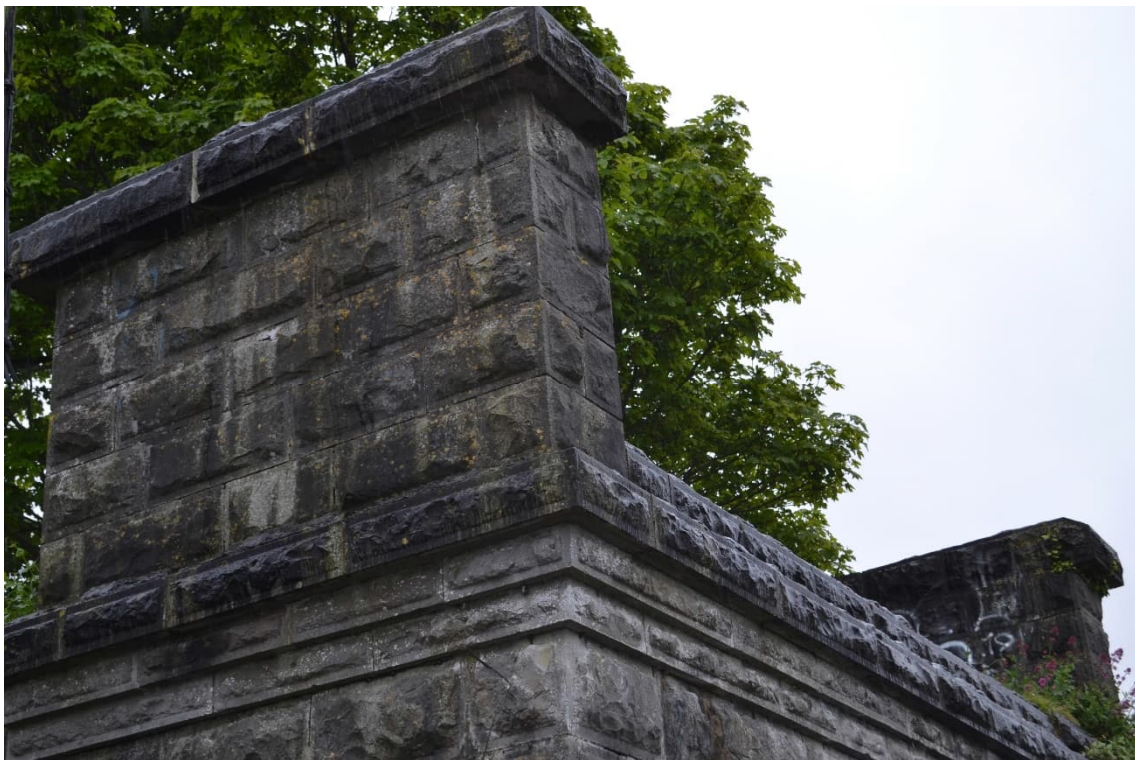
Plate 6 Low walls which flanked the railway roller bearings on the abutment.
