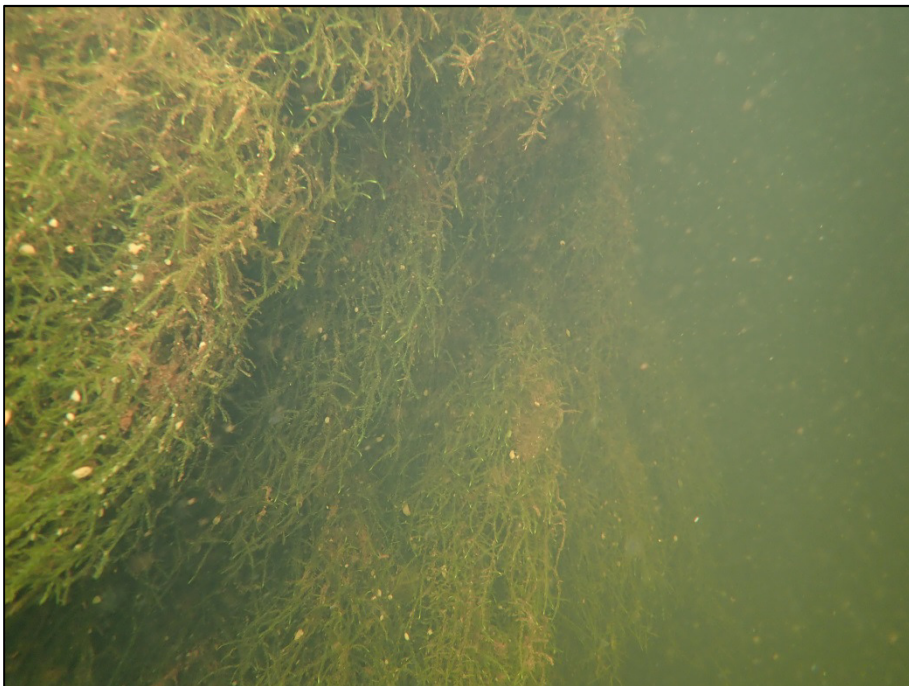
Plate 4: Example shot of riverweed present across the upper parts (first 1.5m-2m) of each of the submerged pier structures.
