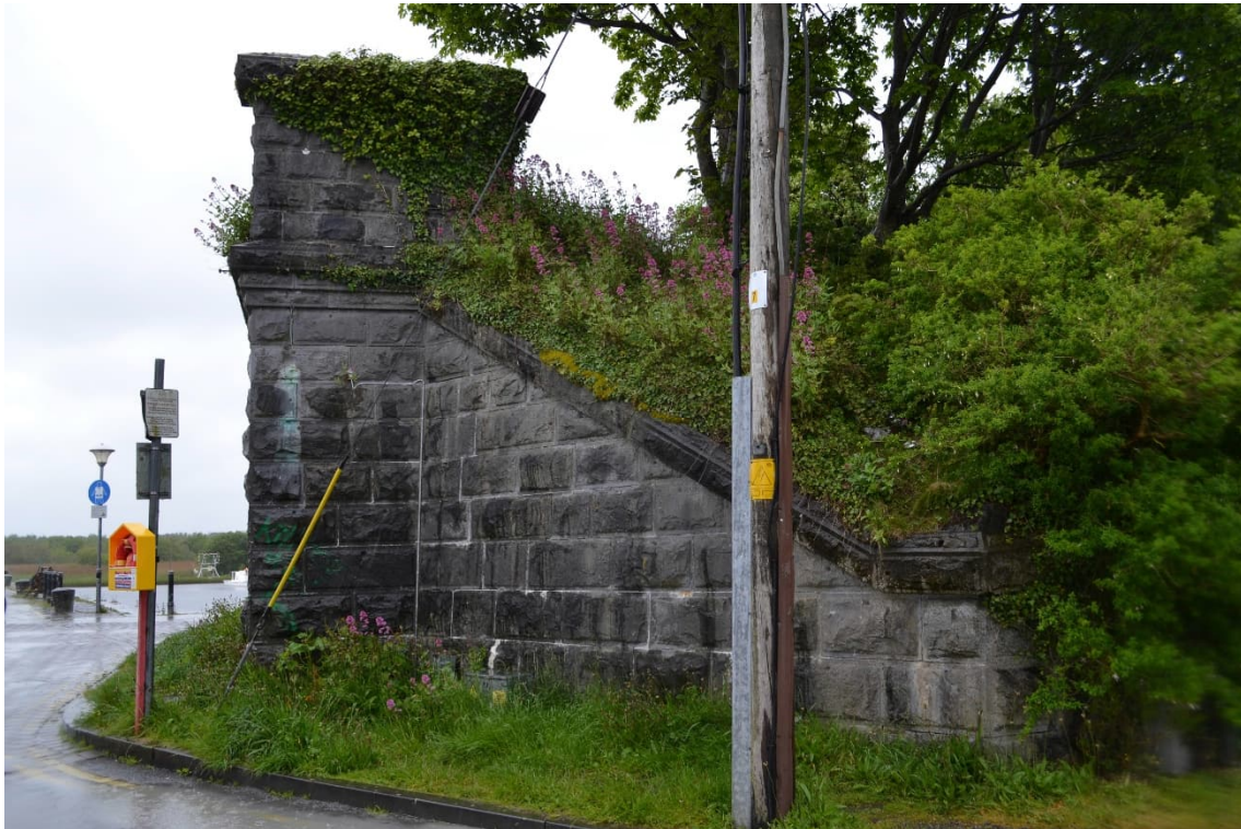
Plate 7 The angled sloping wing wall on the abutment.
