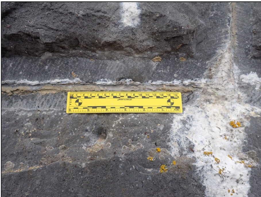
Plate 12: Example shot showing neat/tight seams present between the masonry courses (15mm scale).
