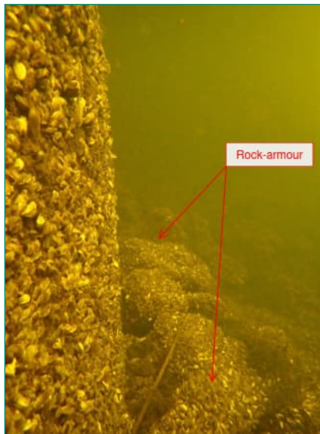
Figure 12-5 Typical underwater view of bridge pier and riverbed including zebra mussel growth
